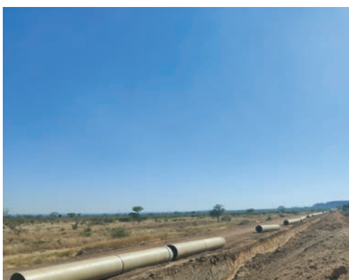
Some of the GRP pipes delivered at the pipeline site at Cowdray Park
