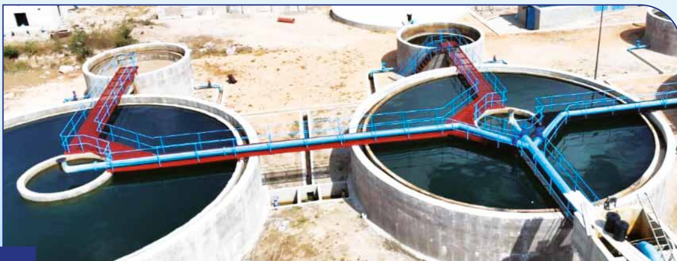
Chivhu Water Treatment Plant
